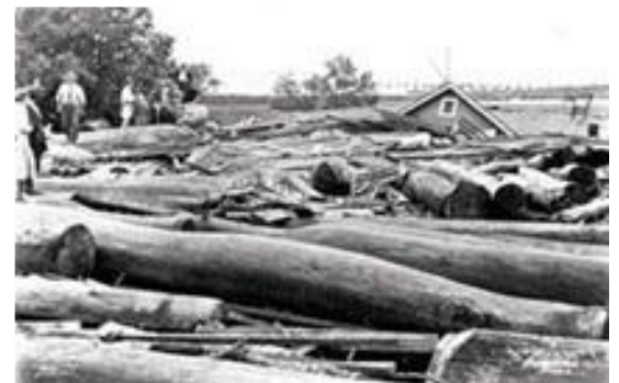
Destruction at Palmetto Beach.*
