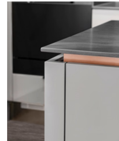
The countertops and backsplash are made of Corian seamless stone, which can effectively prevent dirt and grime, and is easy to clean, maintaining a tidy and hygienic environment. The ripple textures on the seamless stone and the rose gold lining elevate the aesthetic of the kitchen.
