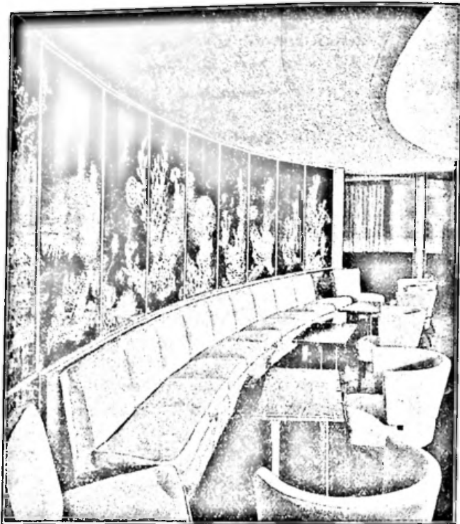
FIG. 20. PARTITION OF CLEAR PLATE GLASS WITH ETCHED DESIGNS
