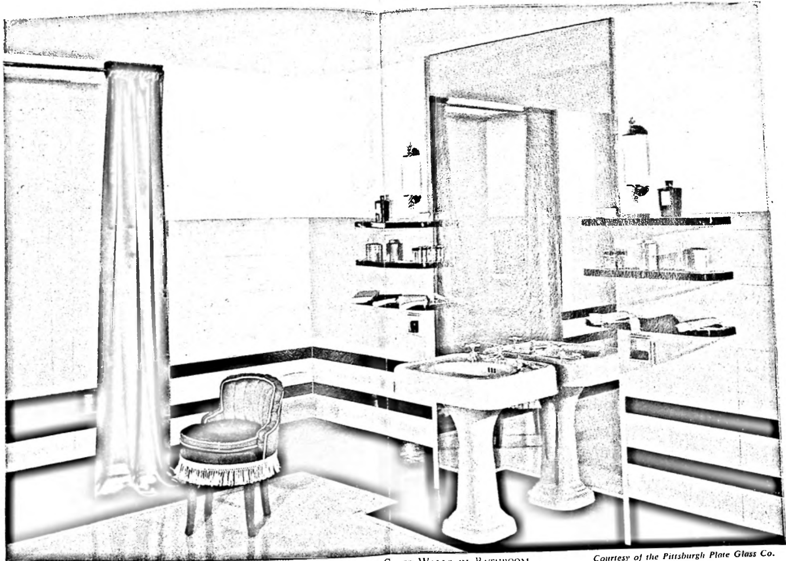
FIG. 18. STRUCTURAL-GLASS WALLS IN BATHROOM
