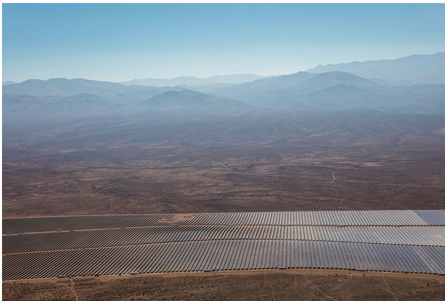
El Romero solar farm in Chile (80 MW for Google)
