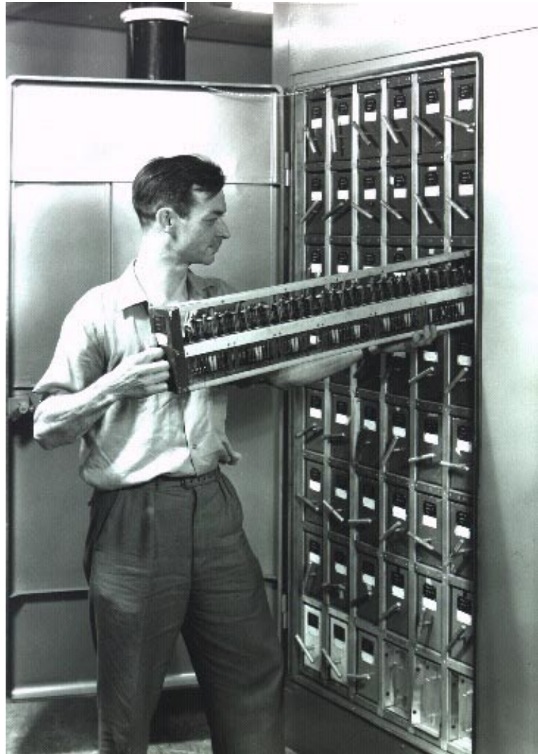
SA Barton & EDSAC 2 chassis construction with miniature valves
