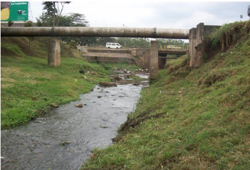
One section of the river reclaimed from the filth
