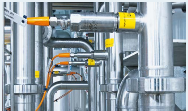
Compact and hygienic: pressure sensor of the PM15 series with flush ceramic measuring cell
