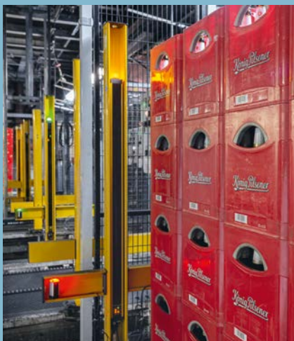
Safety light grid on the pallet lift of a brewery.
