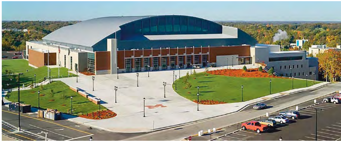
The Mizzou Arena has a large, sloping promenade leading to the entrance doors, rather than stairs.
