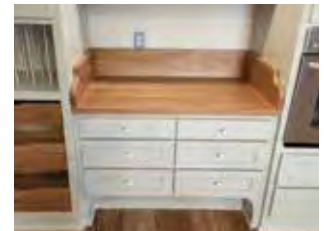
A tall, deep toe kick allows a wheelchair user to get close to the counter.
