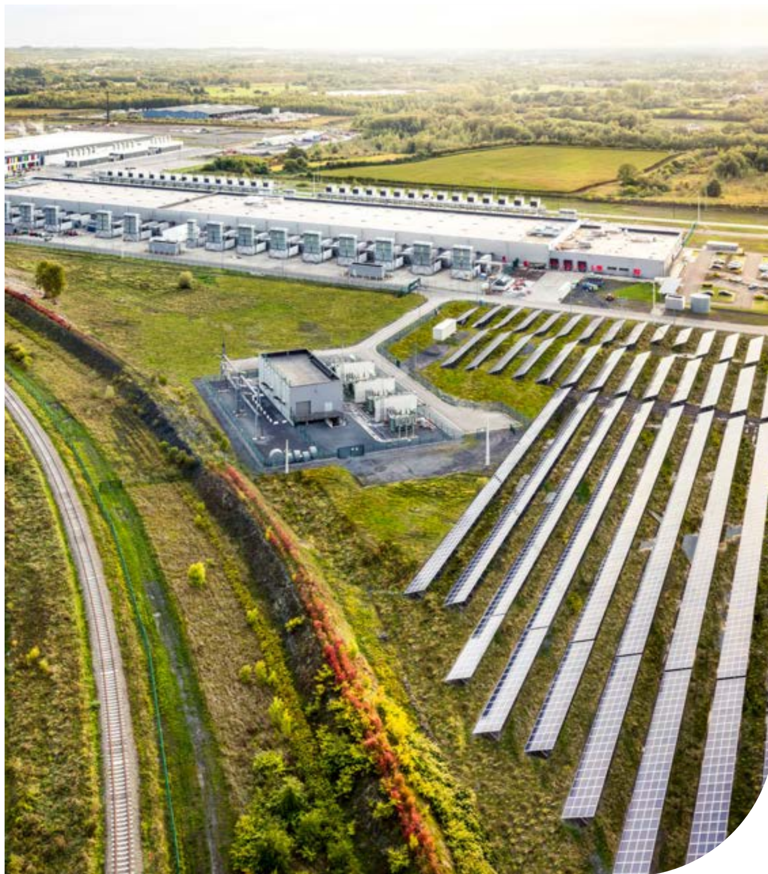
Google's data center in St. Ghislain, Belgium.
