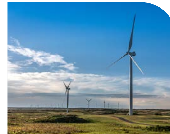
Great Western wind farm in Oklahoma (225 MW for Google)
