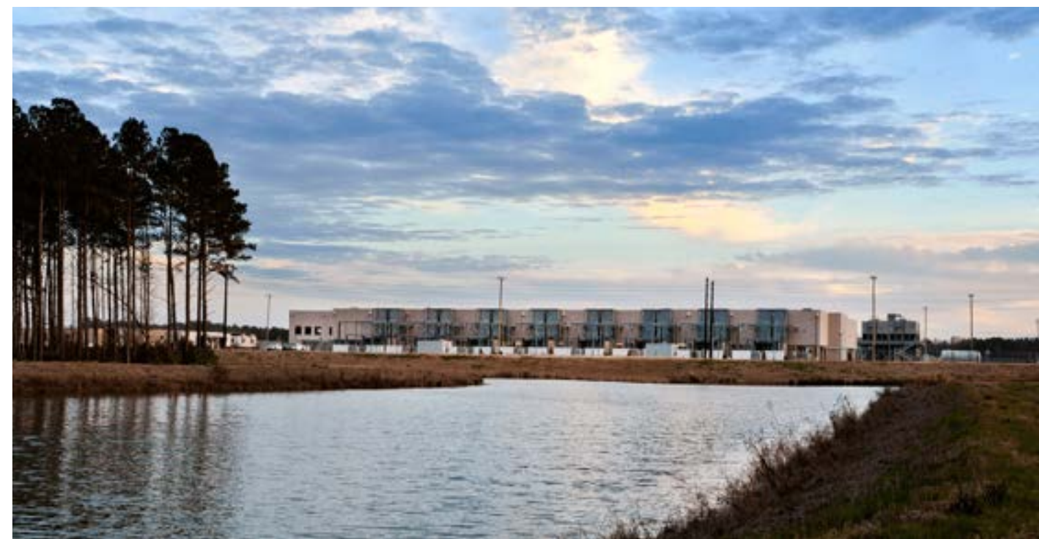
A rainwater retention pond outside our data center in Berkeley County, South Carolina.
