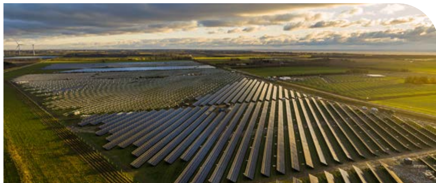
Rødby solar farm in Denmark (55 MW for Google)
