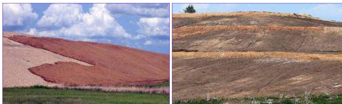
Figure 5. Covering of a stabilized waste rock pile at the mine site No. 9 in N. Kazakhstan
