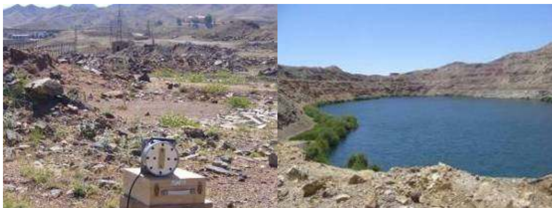
Figure 19. Waste rock piles and former Uranium pit material near former Radium open cast mine covered with water. Contents of dissolved uranium in the water of pit 40-50 Bq l -1 . [15]
