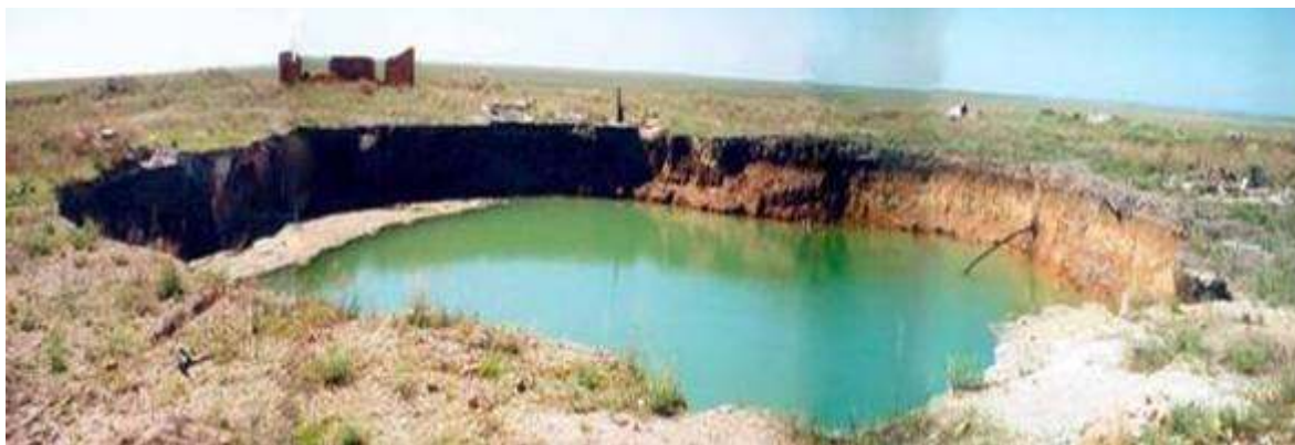
Figure 6. Collapse of the mine No.3 after ground water rebound in northern Kazakhstan
