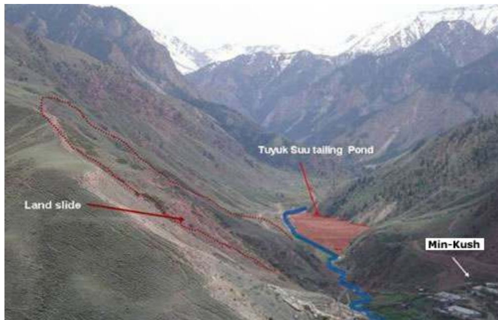
Figure 11. Tailings ponds at the area of Min-ush legacy site and schematic view on the Tuyuk-Suu tailings pond and potential landslide hazard upstream of the Min-kush settlement
