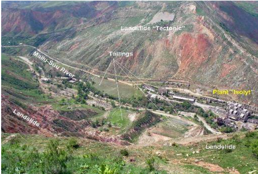
Figure 9. Mailuu-Suu uranium production legacy site and potential main hazards such as landslides
