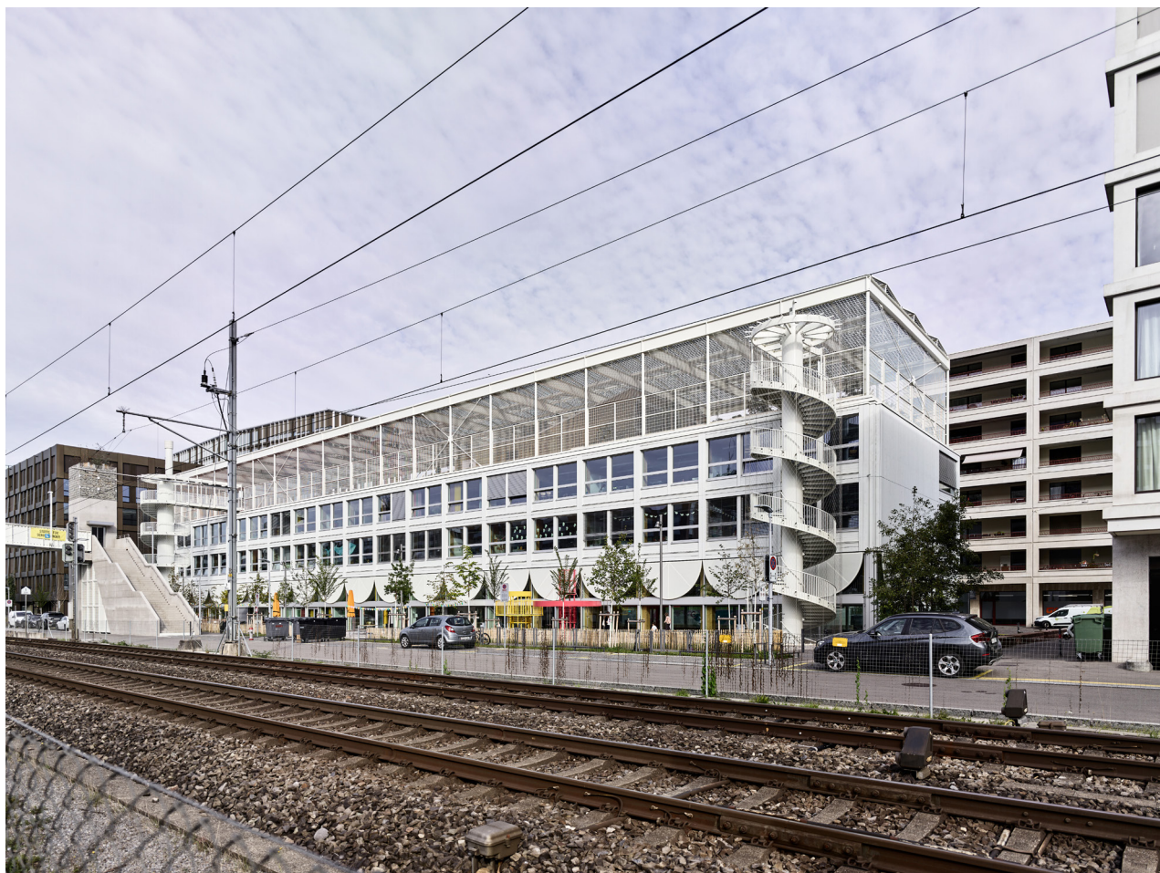
Allmend School in Zürich. Photographer: Matthias Vollmer, Zürich.
