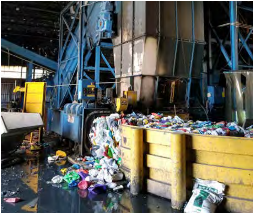
The aftermath of a major fire in May 2023 at the Milwaukee materials recovery facility. While the exact cause of this fire is unknown, a lithium-ion battery is suspected. Photo courtesy city of Milwaukee.
